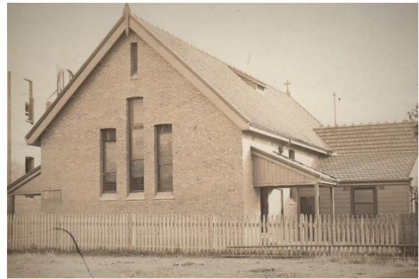
The photo of the 1894 school was taken 1917 as the hall was under construction (on the left).
